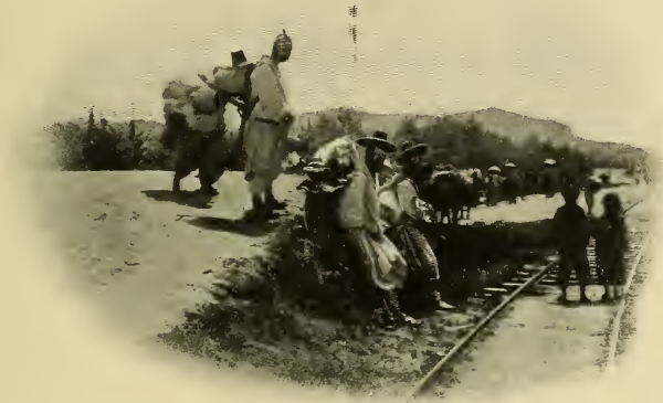
A RAILWAY SIDING
